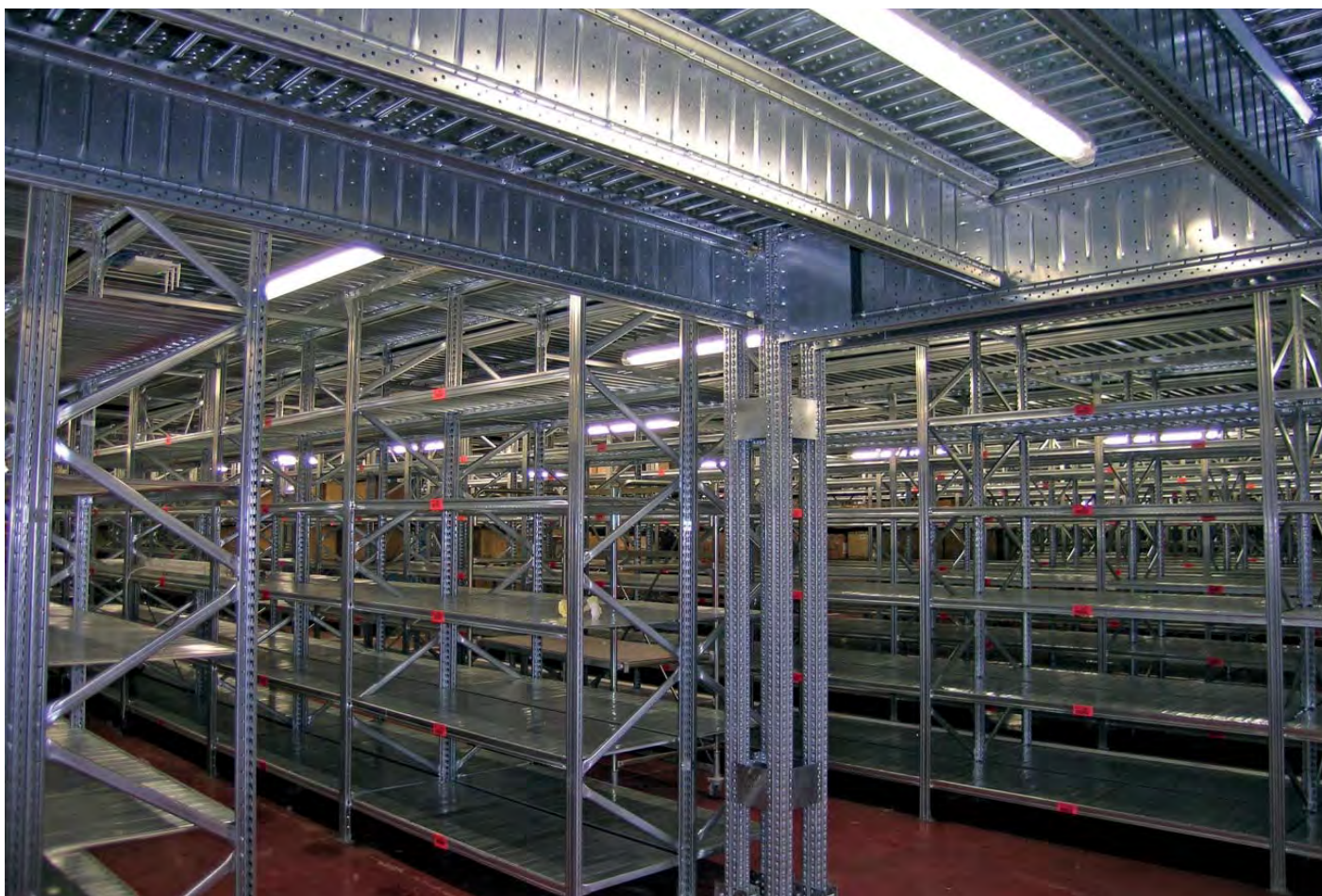
Modular METALSISTEM multi-tier installation and mezzanine made from METALSISTEM's UNIRACK and SUPER-6 product series <Handover in June 2012>
