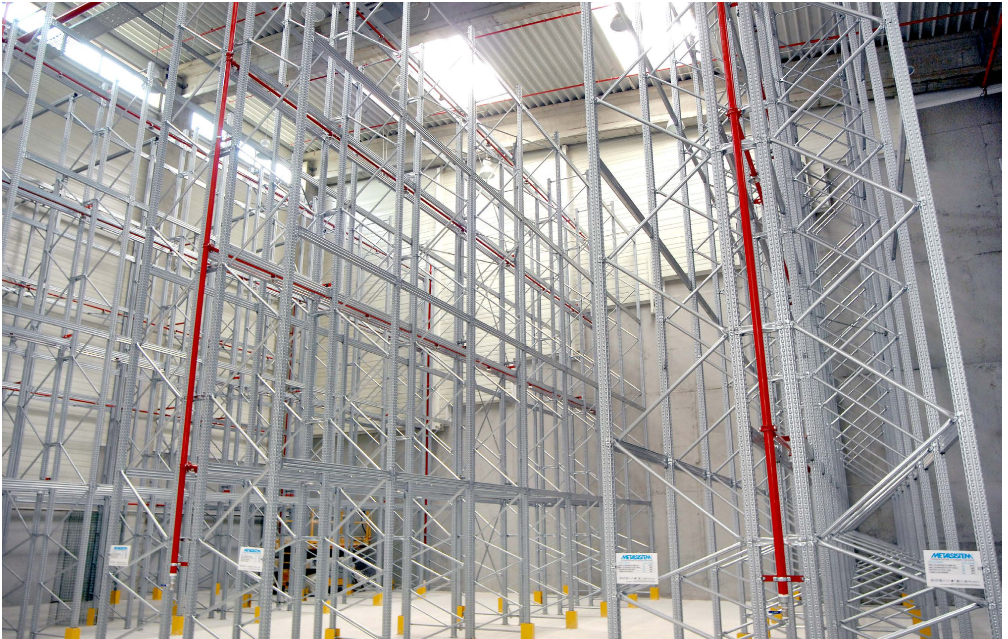
Super 4-5-6 Pallet racking installation. <September 2013>
