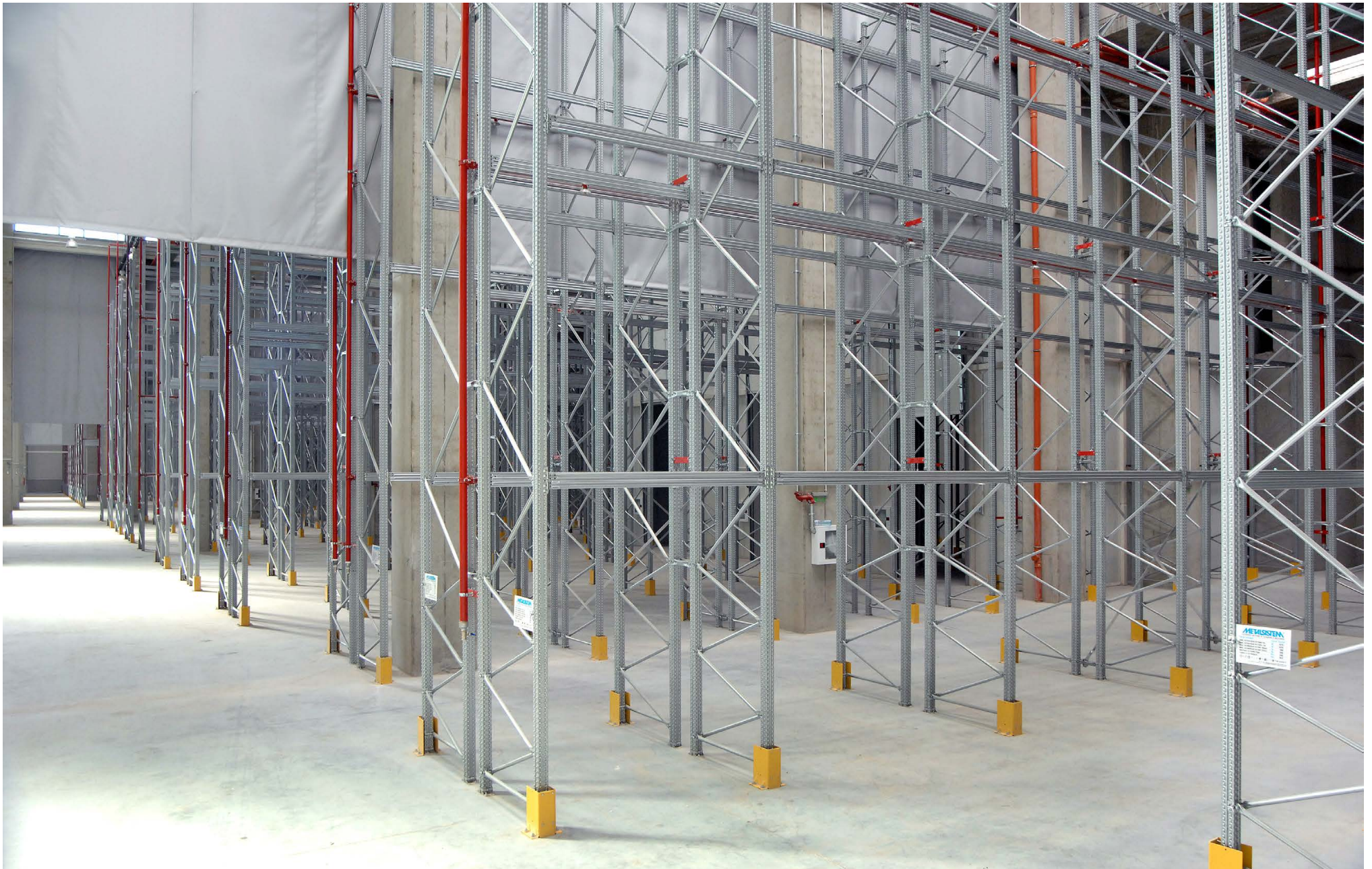
Super 4-5-6 Pallet racking installation. <September 2013>
