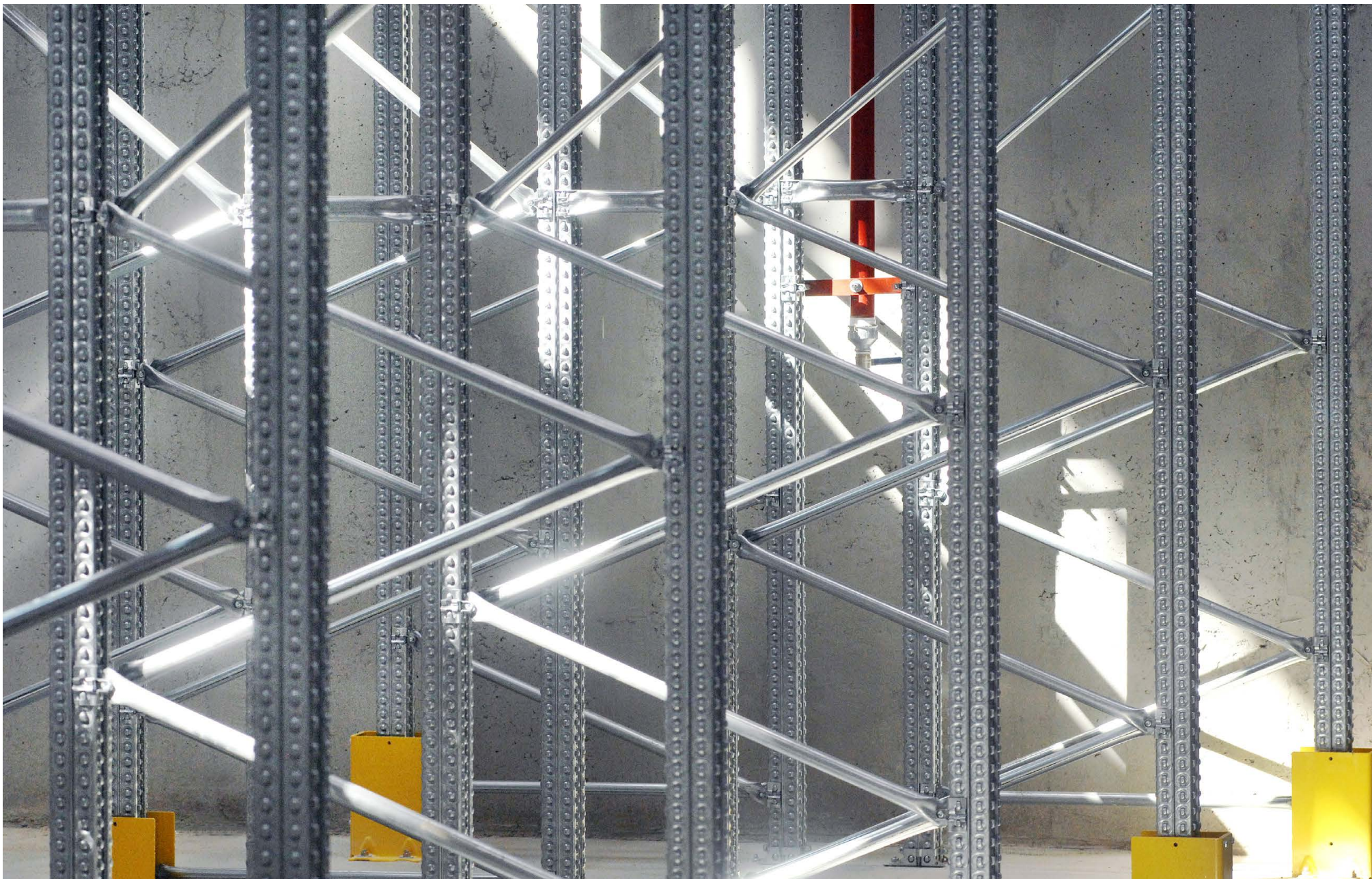
Super 4-5-6 Pallet racking installation. <September 2013>
