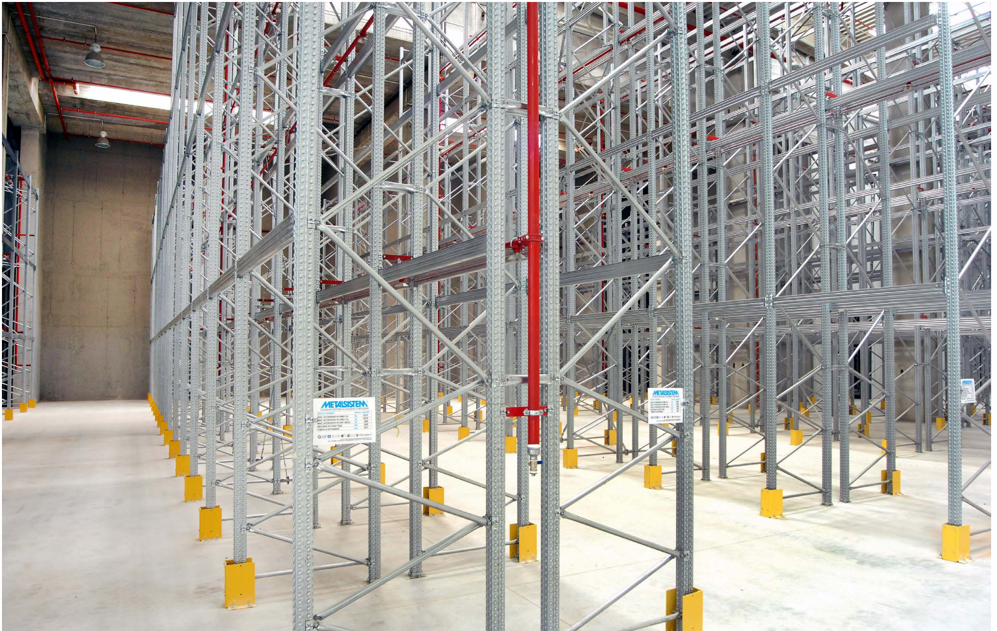
Super 4-5-6 Pallet racking installation. <September 2013>
