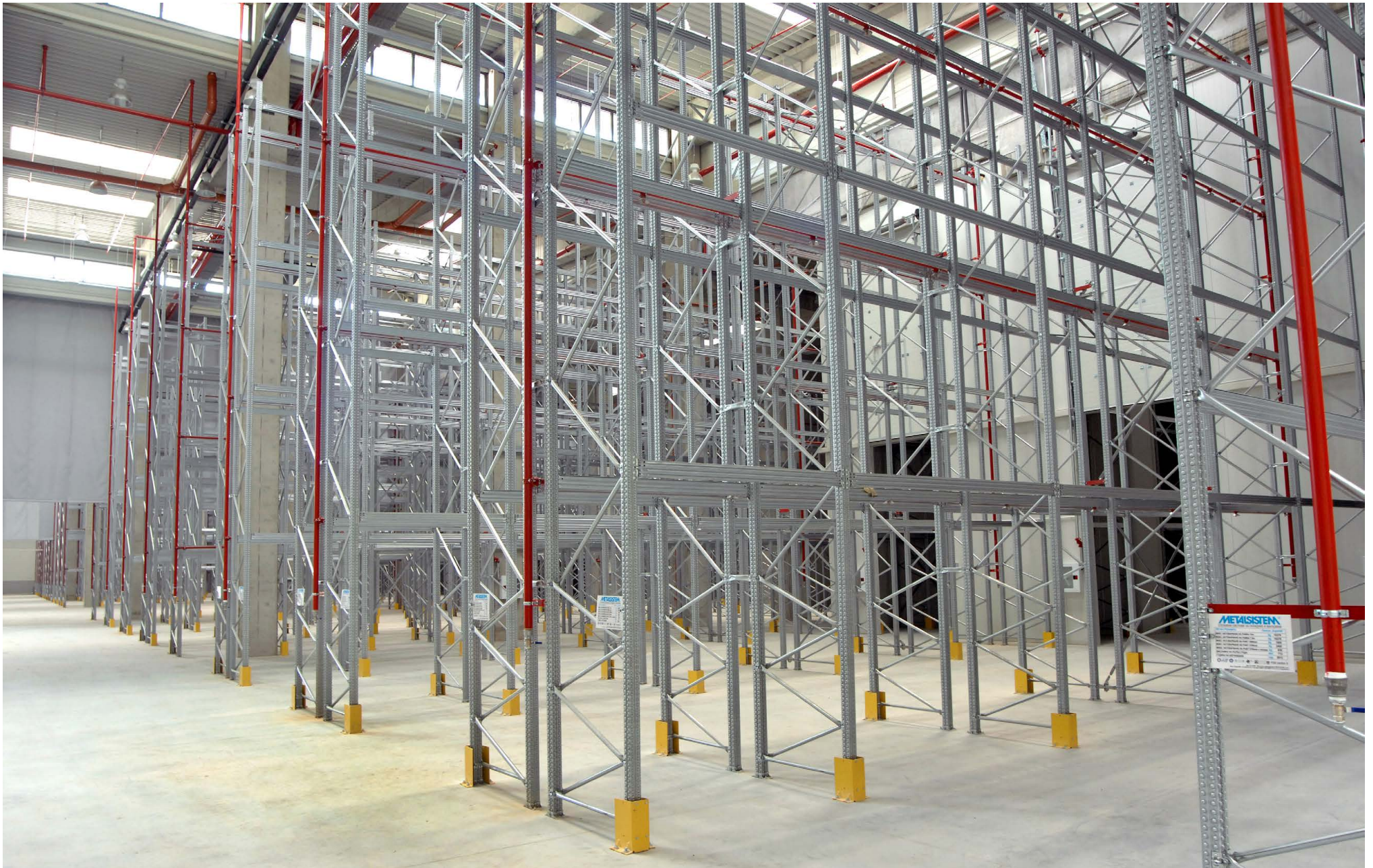
Super 4-5-6 Pallet racking installation. <September 2013>
