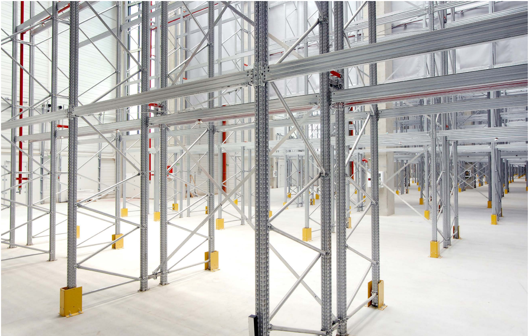
Super 4-5-6 Pallet racking installation. <September 2013>
