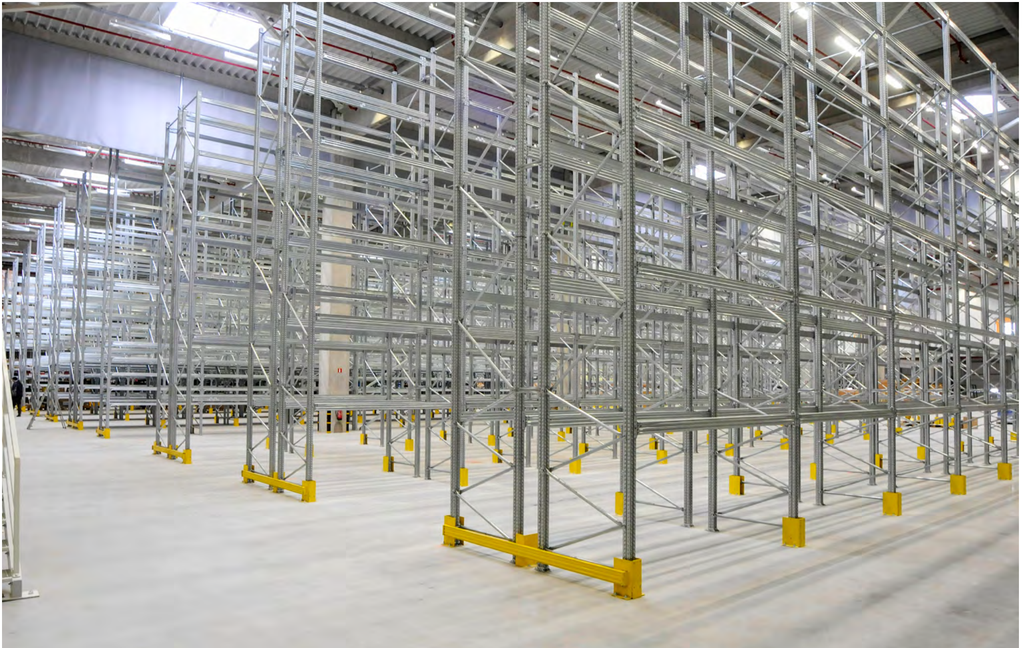
Super 6 - Pallet Racking Reference Installation <April 2015>
