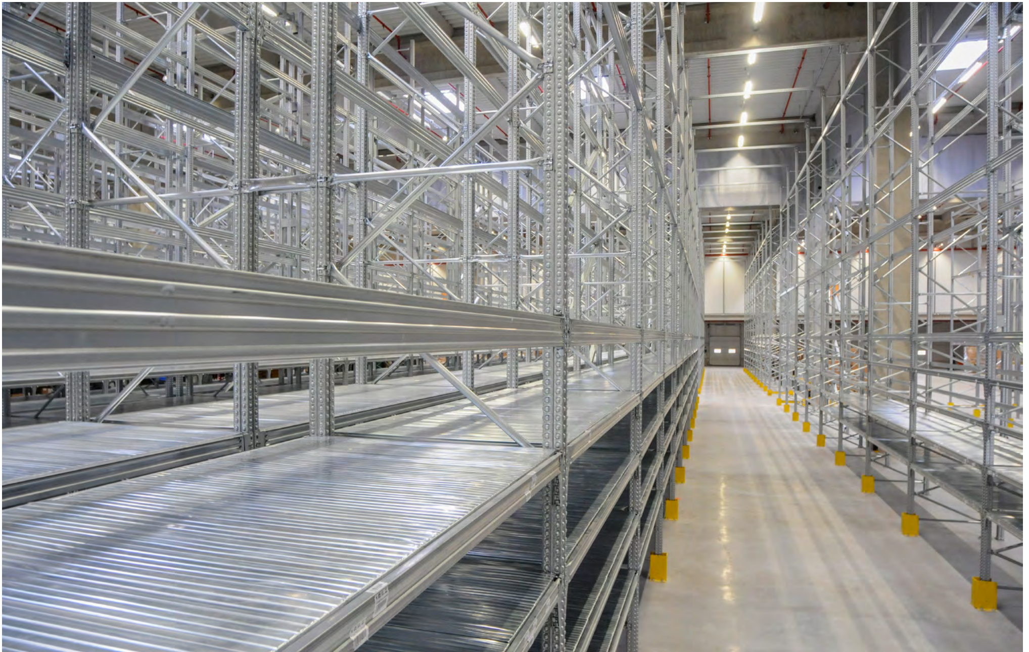
Super 6 - Pallet Racking Reference Installation <April 2015>
