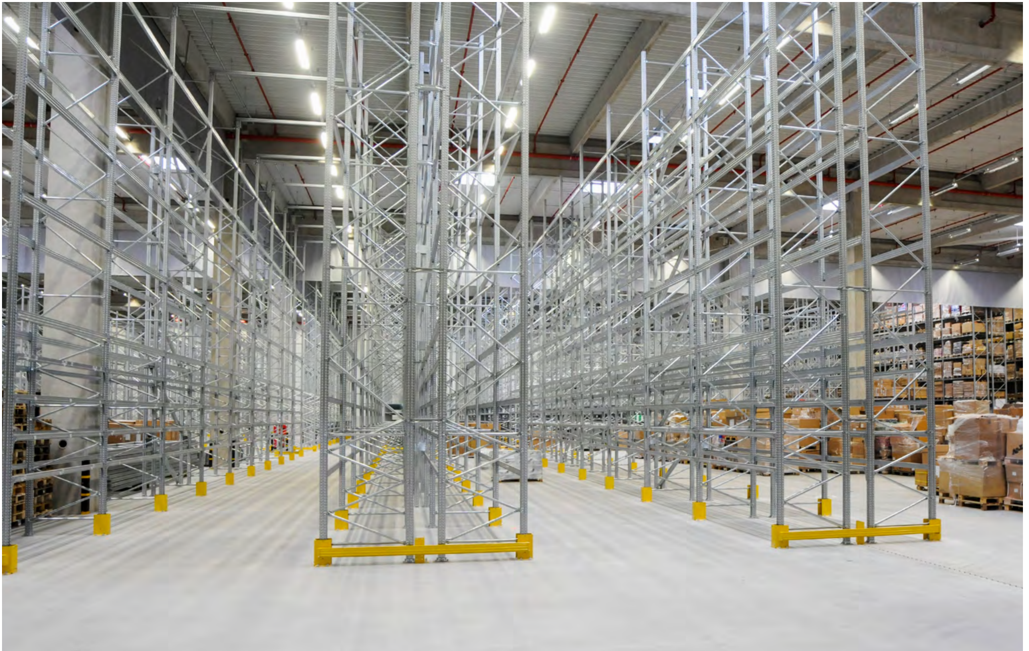
Super 6 - Pallet Racking Reference Installation <April 2015>
