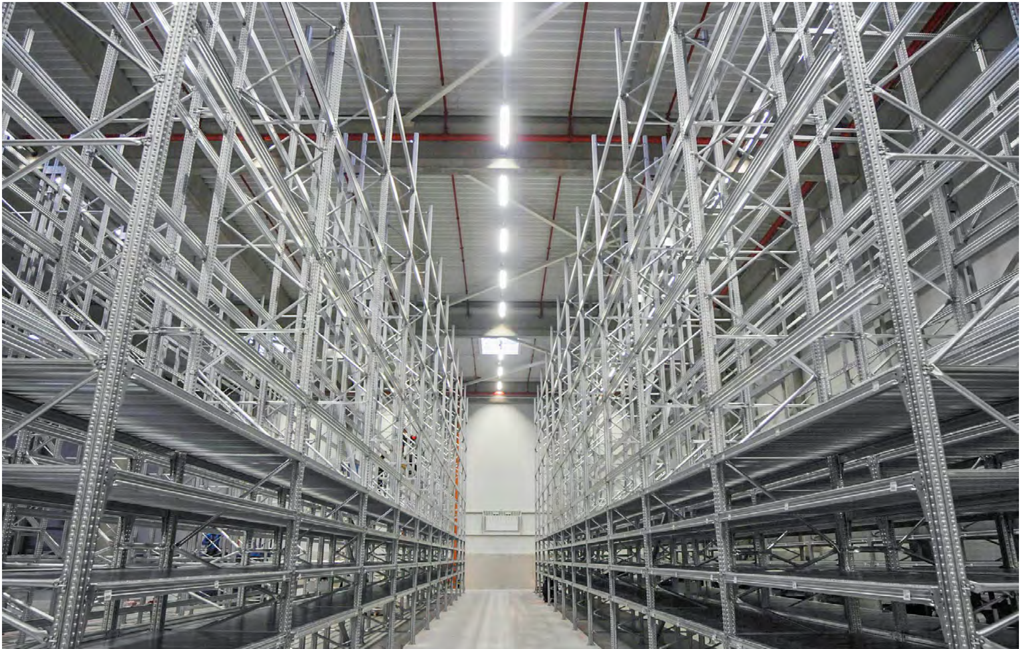
Super 6 - Pallet Racking Reference Installation <April 2015>
