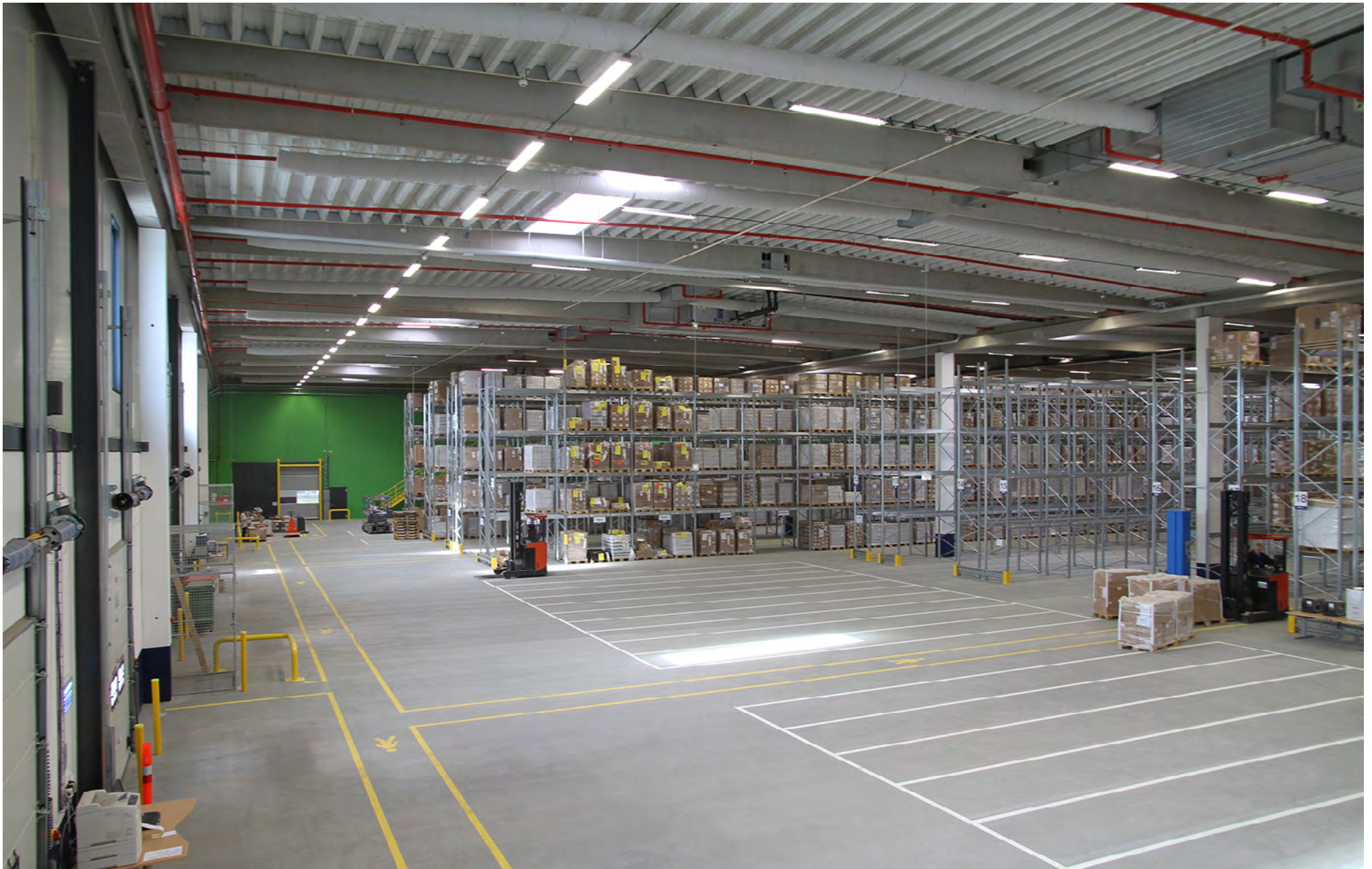
SUPERBUILD - Pallet Racking Reference Installation - Pharmaceutical Products.
